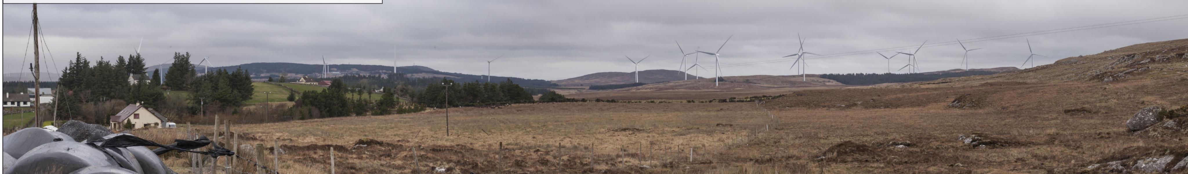
Proposed Option 2: 11 Enercon 138 Turbines: Hub Height: 81m, Rotor Diameter: 138m, Tip Height: 150m.
