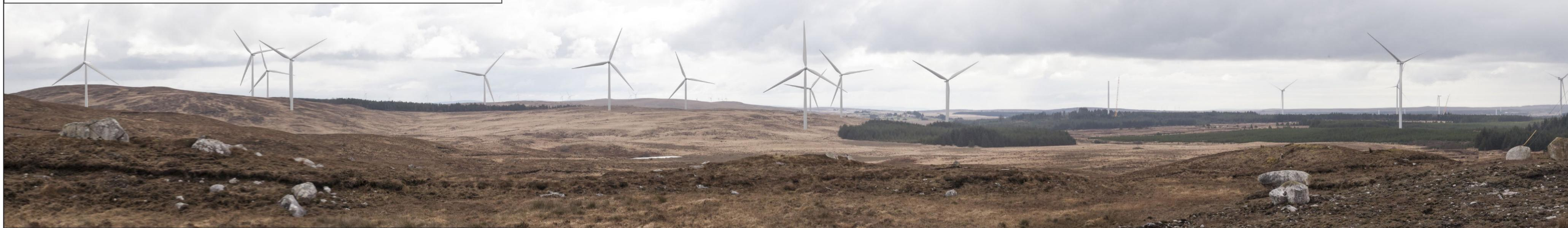
Proposed Option 2: 11 Enercon 138 Turbines: Hub Height: 81m, Rotor Diameter: 138m, Tip Height: 150m.
